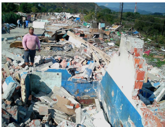
Demolition in progress
